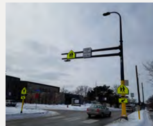
Traffic control device and APS push buttons
