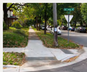
ADA-Compliant Curb Ramps
